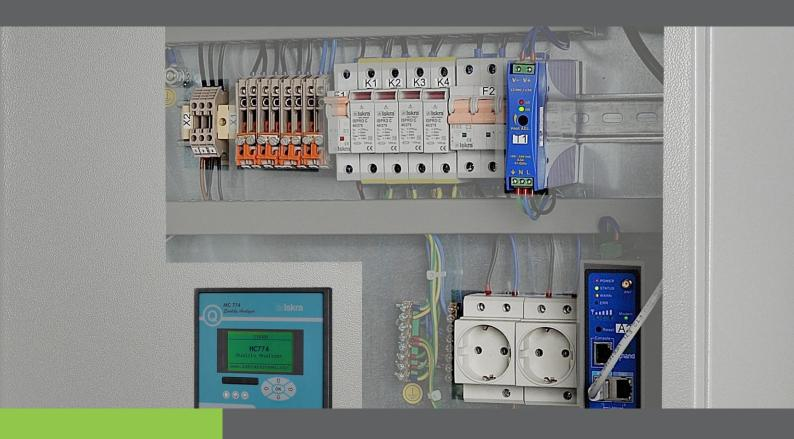
Integrated Metering Cabinet for Remote Energy System Monitoring
